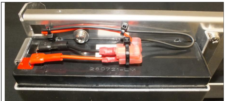
Figure 6: Bundling using cable ties
